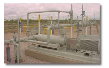
Installation Location: West Texas Pump Model: DLH12DHT-400 Rotating Speed: 1750 rpm System Pressure: 1000 psig Flow Rate: 400 gpm Fluid: Light Crude Oil
