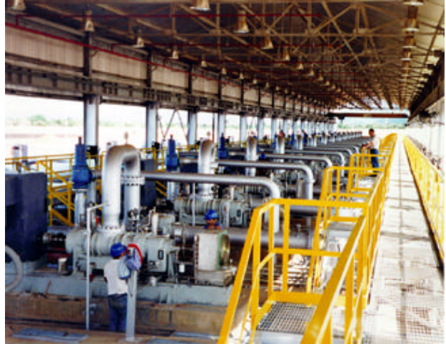
Figure 7 – 15 Twin Screw Pumps for SUBSEA Pipeline
